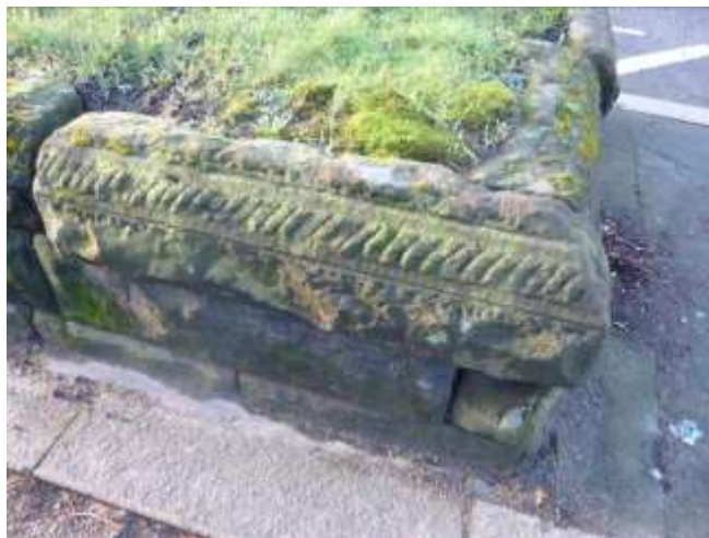
Retaining wall to Manchester Road central island
