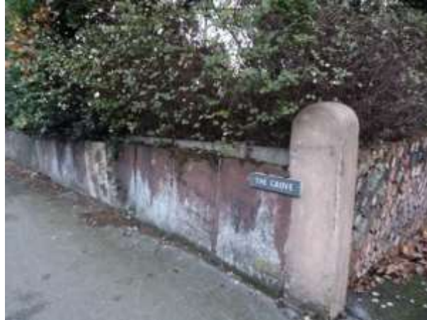
Stone flags used as a boundary treatment to land occupied by The Grove
