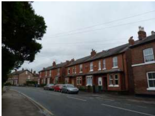
Nos. 28-42 (even) Oldfield Road
