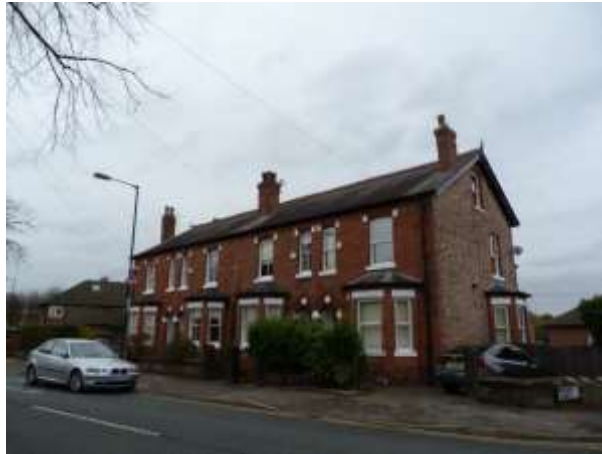
Nos. 44-50 (even) Oldfield Road
